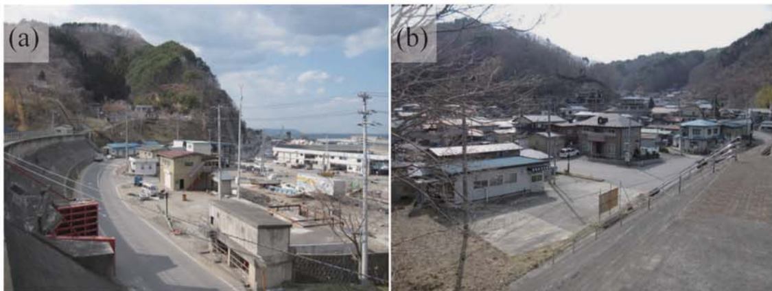
Fig. A48. (a) Destructive damage outside the coastal levee (Otanabe Fishing Port). (b) Very minor damage inside the coastal levee (residential district). (c) Tsunami trace survey point at the name board of the fish market (I22) (d)-(e) Watermark on the wall of a hair salon (2.2 m above ground level; I23). (f) Tsunami trace survey point at the middle of the coastal levee (I24) (g) Tsunami trace survey point at the middle of the coastal levee (I25).
