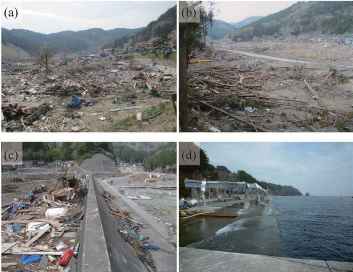
Fig. A122. (a)-(c) Damage at Hongo. (d) Subsidence of a wharf at Toni Fishing Port. (e) Tsunami inundation limit at a slope beside a house in the northern area of Hongo (I124). (f) Fishing net and debris caught on a branch of a tree (5.61 m above ground level, I125). (g) Tsunami trace survey point at a garden on the north-side slope (I126). (h) Tsunami inundation limit in a forest on the southern slope (I127). (i) Tsunami inundation limit on the southern slope judged from the end of a pile of debris (I128).
