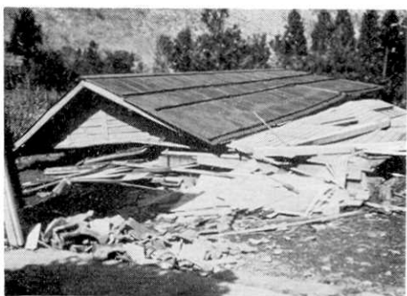
Fig. 19. Total failure of storage shed.
