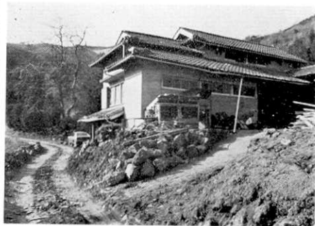
Fig. 54. Damage to stone retaining wall and house at Uchiyama village.
