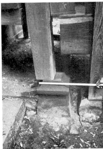
Fig. 27. Column dislodged from footing.
