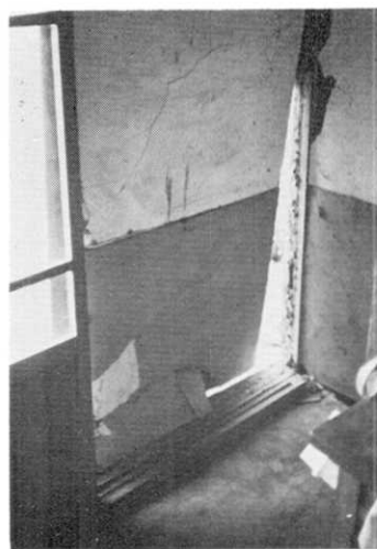
Fig. 16. Separation of mud wall by the entrance.
