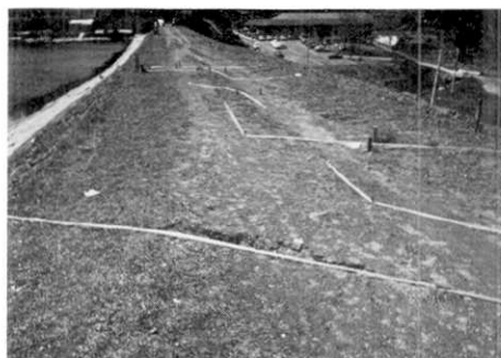
Fig. 49. Cracks on the surface of the crest of Yamashita-Lake dam.
