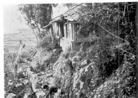
Fig. 28. House damaged due to failure of masonry retaining wall.
