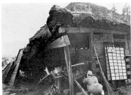
Fig. 11. Total destruction of shed due to failure of stone retaining wall.
