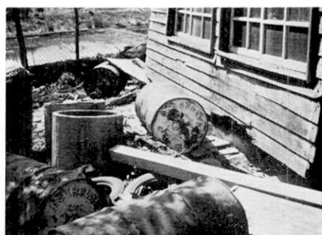
Fig. 18. Separation of shed from wall foundation.
