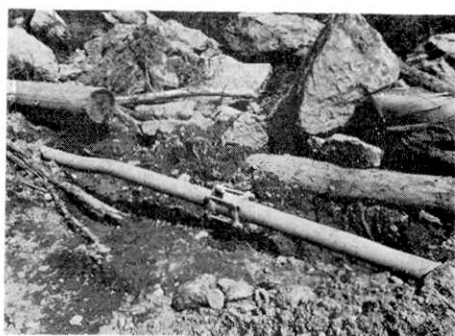
Fig. 50. A new water pipe which is replaced with the old one crushed by fallen stones.
