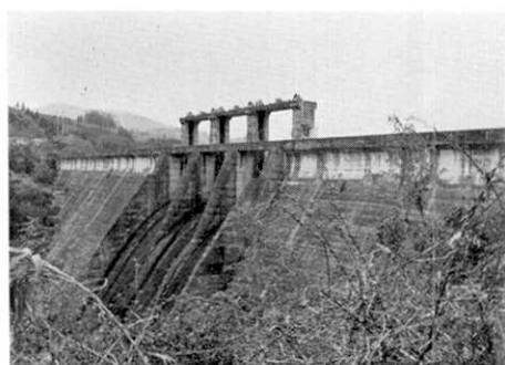
Fig. 45. Serikawa gravity-type concrete dam. (No damage was discovered.)
