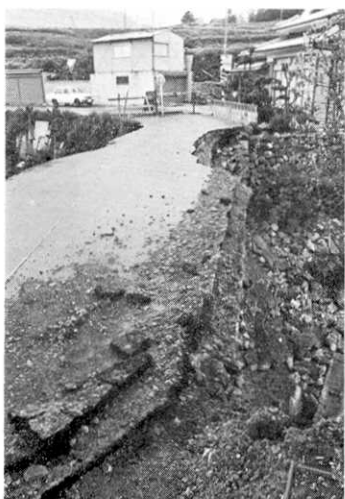
Fig. 42. Damage to spandrel stone masonry of Kōno stone arch bridge.
