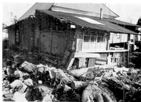
Fig. 53. Damage to stone retaining wall and house at Uchiyama village.
