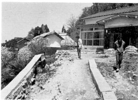
Fig. 52. Damage to masonry retaining wall at Okunameshi village.
