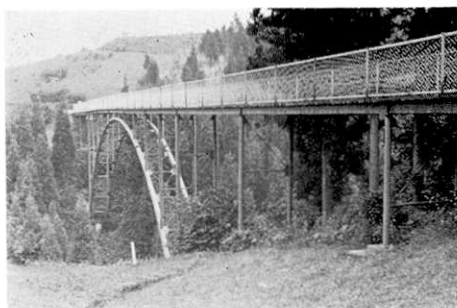
Fig. 44. Rising of floor deck by 16.5 cm of pipe-arch bridge.
