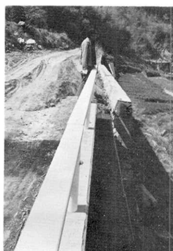
Fig. 43. Swelling of masonry retaining wall and settlement of soil behind bridge abutment.
