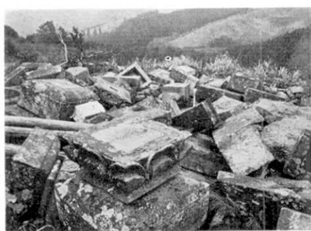
Fig. 61. Graveyard at Shiode. All gravestones fell to the north or south.
