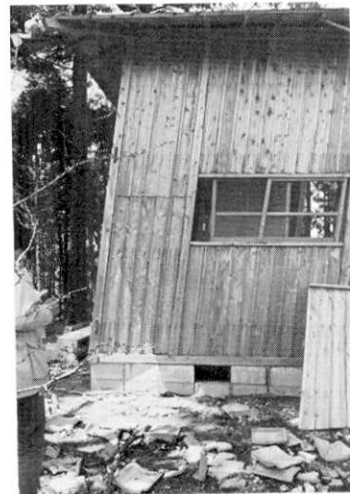
Fig. 26. Tilted unbraced hut.
