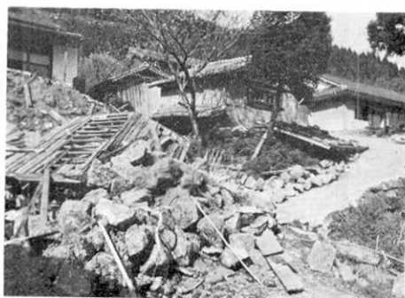
Fig. 55. Damage to stone retaining wall at Uchiyama.
