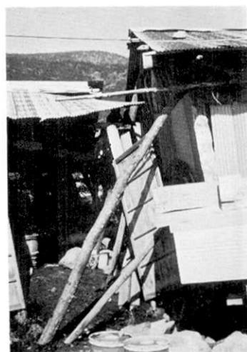
Fig. 14. House tilted, due to poor construction.
