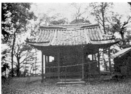
Fig. 29. Damage to roof ridge tiles of a shrine.
