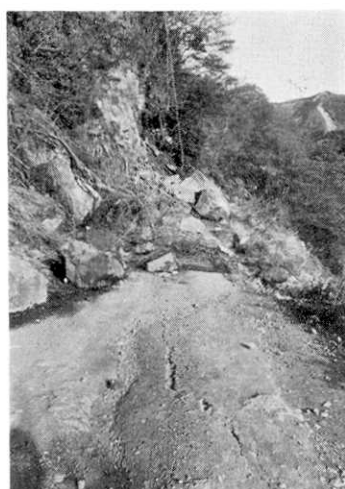
Fig. 32. Slidden deposit on a road from cutting slope.
