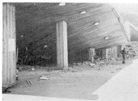
Fig. 21. Slightly damaged long columns.
