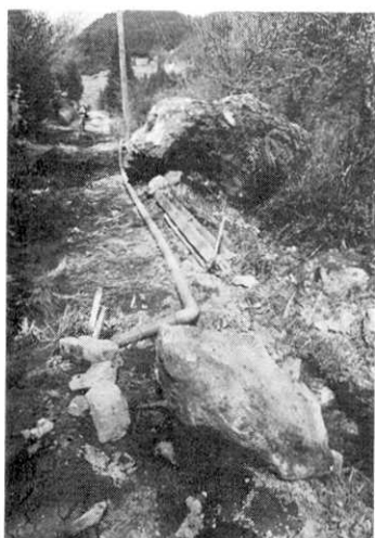
Fig. 33. Fallen stones on a road which destroyed a water pipe buried 50 centimeters below the surface of the ground.
