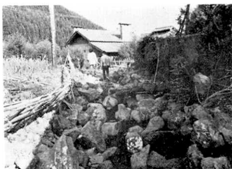
Fig. 56. Damage to stone retaining wall at Uchiyama.
