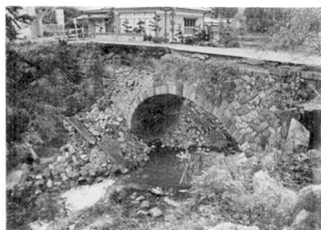
Fig. 41. Damage to spandrel stone masonry of Kōno stone arch bridge.
