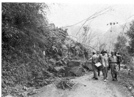
Fig. 31. Slidden deposit on a road from cutting slope.
