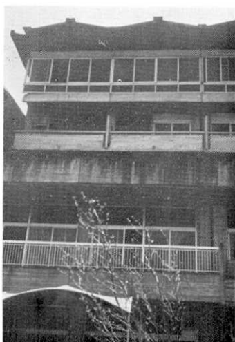
Fig. 22. Pounding of expansion joint.
