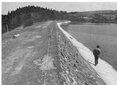
Fig. 48. Yamashita-Lake earth dam. There were many cracks in the stone pitching.
