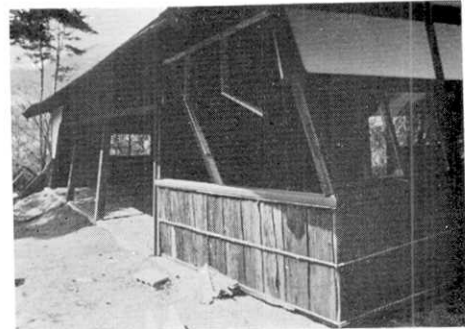
Fig. 24. Failure of open frame viewing hut.
