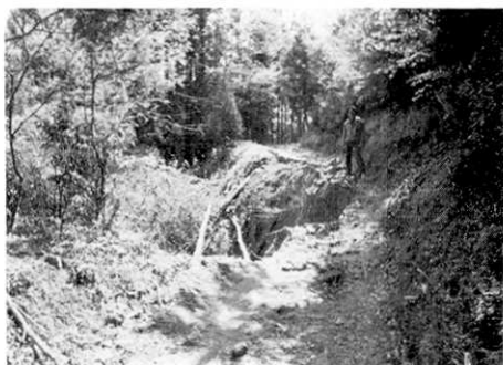
Fig. 35. Slope failure of embankment.
