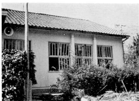
Fig. 17. Deformation of window.
