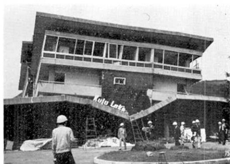
Fig. 20. Partial collapse of ground floor of Lake Side Hotel.
