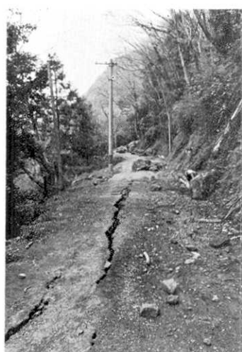
Fig. 34. Cracks on road surface.
