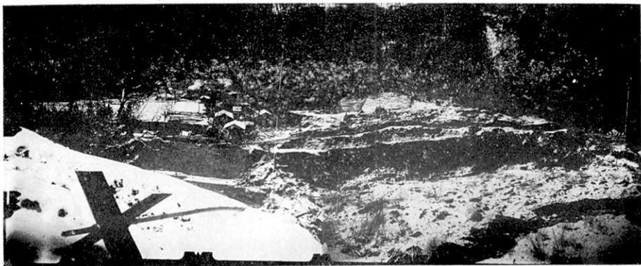
b. The mud flow flowed down the slope across the river in the foreground and leaped over the road and destroyed and buried a house standing at the higher level. The present road runs on the debris.
