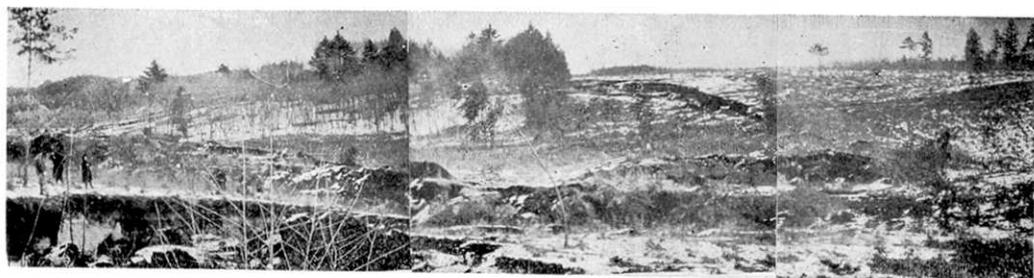
a. Low angle landslide at Tsuchizawa, Imaichi Town. Land before the crack fissure in the central part slid bodily with forest almost undisturbed. The ridge in the foreground is the result of upthrust at the margin of the slid land.
