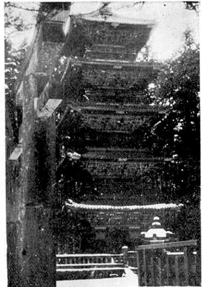
d. The pagoda suffered no damage. The upper part of *torii* (above the crack) was twisted a few cm.
