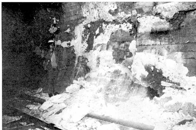
Fig. 25. Exfoliation of the concrete lining of the tunnel.
