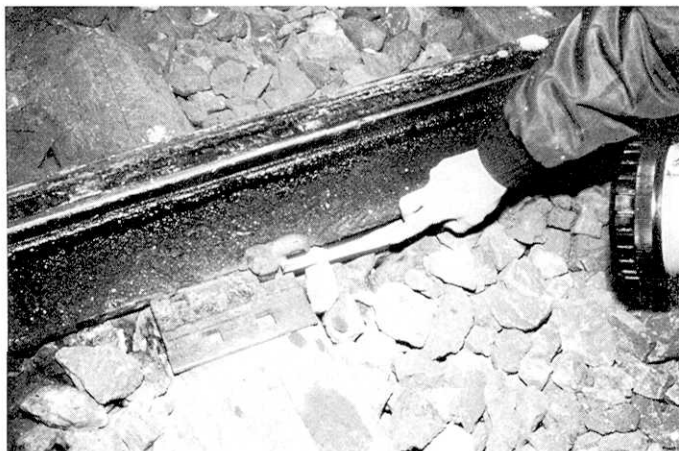
Fig. 29. Slipping of a rail on the tie-plate as revealed by the scratch of the dog-spike on the flange of the rail.
