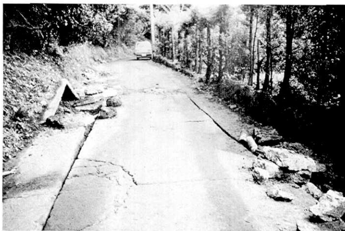
Fig. 15. Roadside concrete slab rotated and buckled in a chevron shape and the central main slab rotated in a clockwise sense (Loc. E-2).
