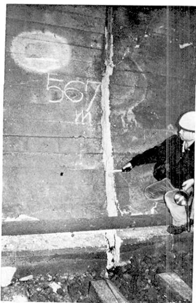
Fig. 27. Open crack on the side wall of the tunnel.
