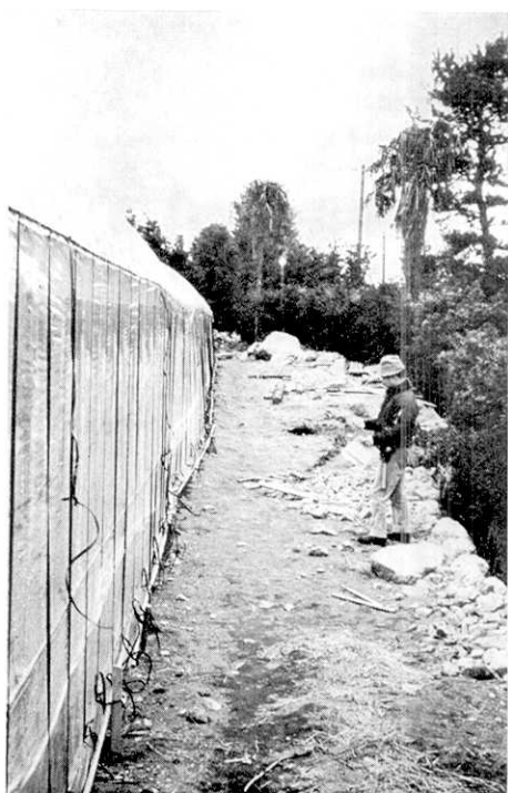
Fig. 18. Displaced wall a-b of the hothouse shown in Fig. 17.
