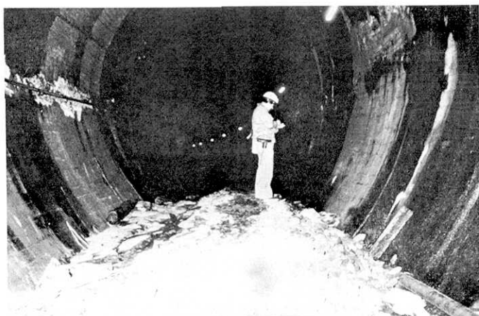
Fig. 26. Squeezing up of ballast due to lateral pushing of the side wall of the tunnel.
