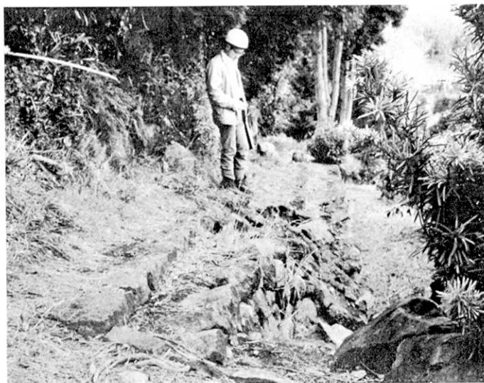
Fig. 16. Displaced stone wall in an orange field (30 m northwest of Loc. P-1).
