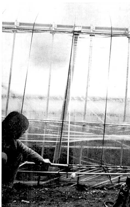
Fig. 19. Close view of one of the hothouse's pillars leaning away from a vertical position (Loc. I-2).
