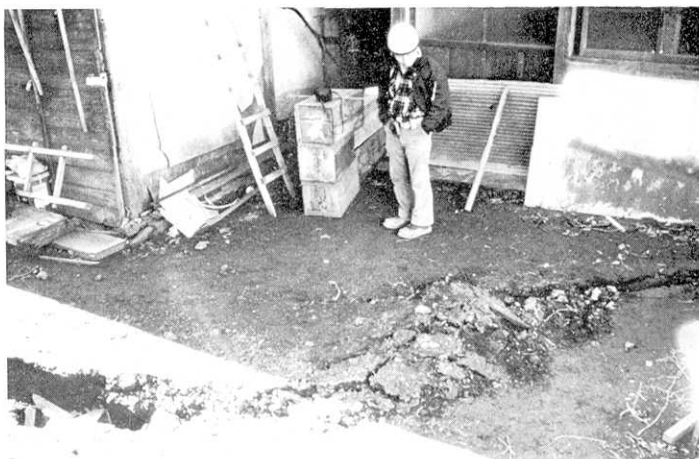
Fig. 6. Pressure ridge formed between adjacent en-échelon ground cracks (Loc. F-2).
