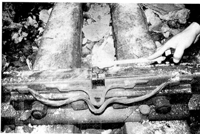
Fig. 28. Abnormally enlarged joint clearance.
