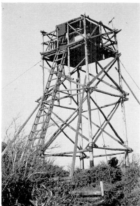
Fig. 3. Instrument station of the Togasayama base-line network (top of Mt. Togasayama).
