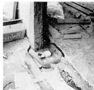
Fig. 1e. Lateral sliding of a house on the foundation at Kami-sagano.
