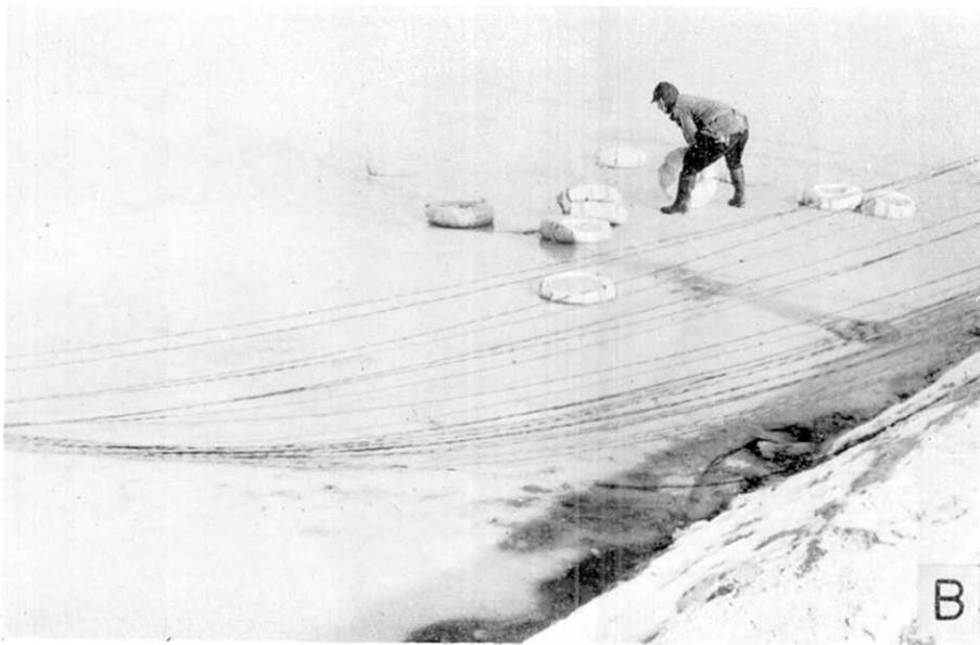
Cables that connect detectors to the recording equipments.
