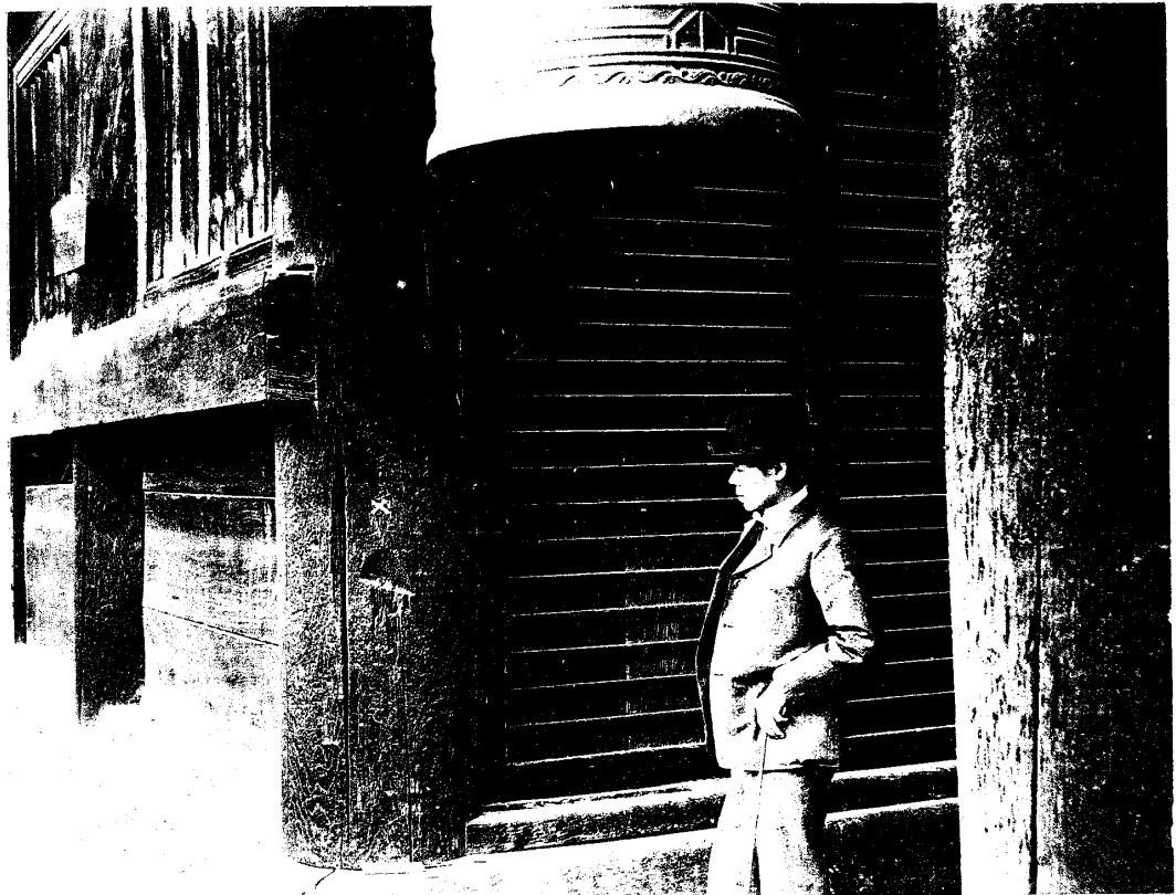
Fig. 3. The Zenkoji Temple, showing the scar (indicated by a small cross x) made on the corner post by the bell thrown down on the occasion of the earthquake of 1847.
