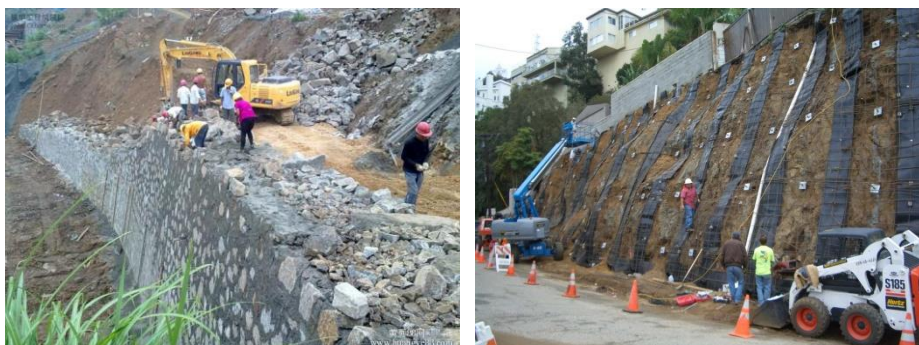
Figure 1.1: Typical landslide protection works; (a) retaining wall, (b) soil nailing
