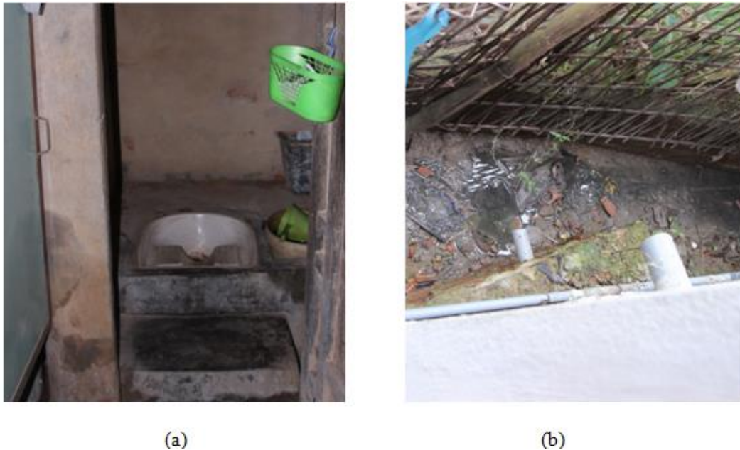
Figure 12 - Typical Household pour-flush pit latrine (a); Blackwater overflow and gray water discharged to backyard (b) (Photo taken by Author)
