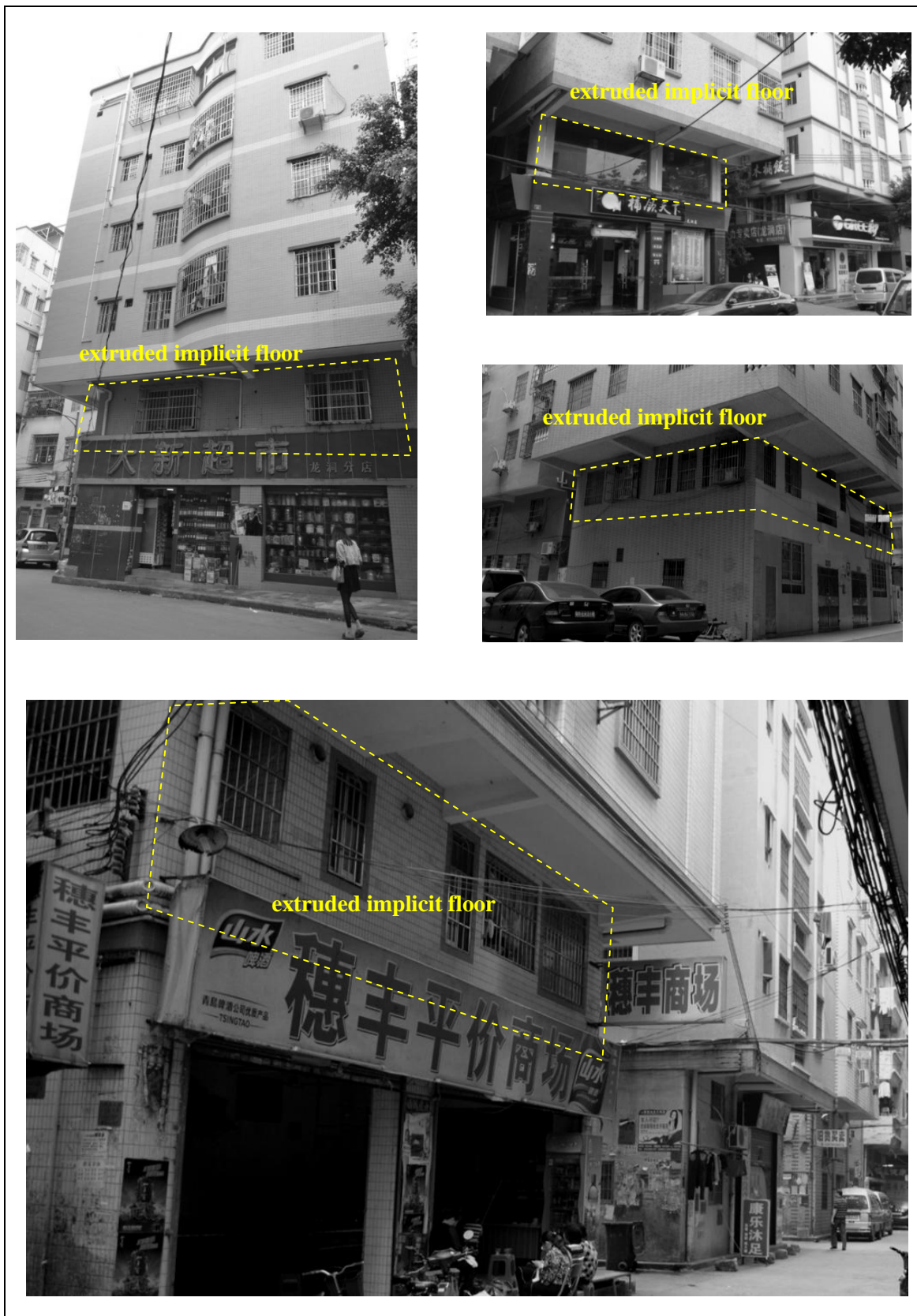
Fig. 182 Cases of the extruded implicit floor above 1 st floor in Longdong Village, Guangzhou Source: by author in 2013
