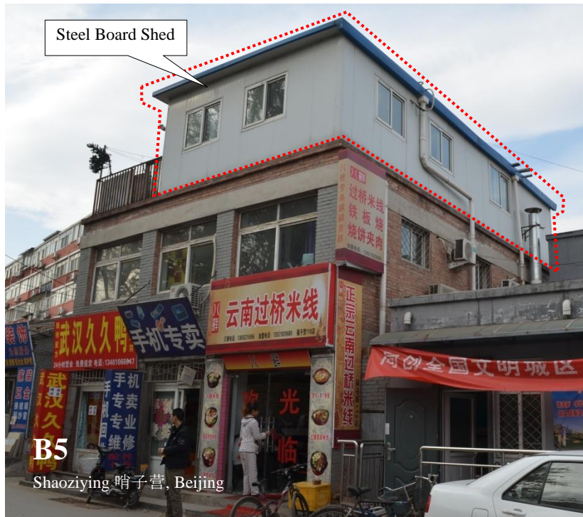
Fig. 188 Case of addition on existing house in Shaoziying, Beijing Source: by author in 2012
