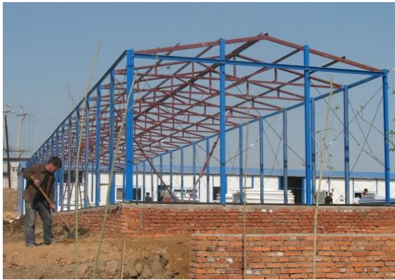
Fig. 183 Light steel structure of Caibanfang
