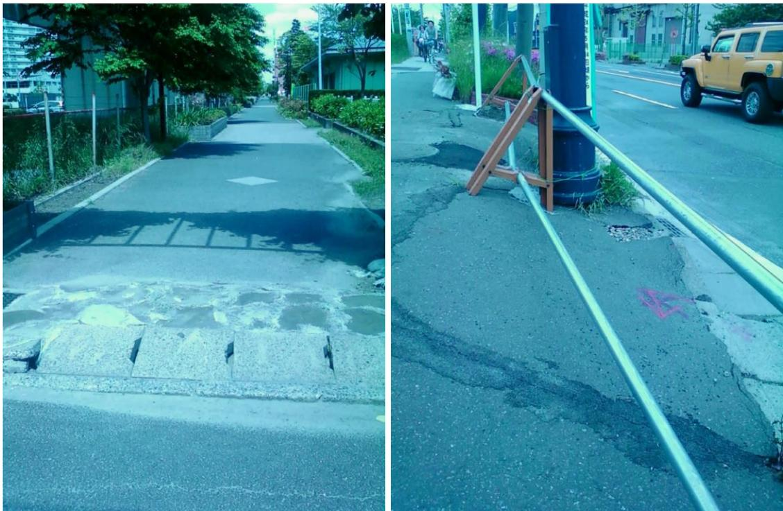
**Figure 2.12. Liquefaction on the streets**
