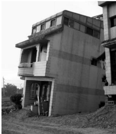
**Figure 2.4. Liquefaction-induced tilting in a residential building (from Hung 2012)**
