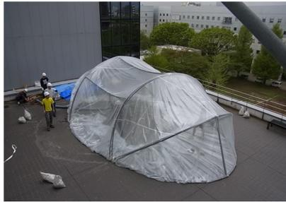
Fig.7-19 New folding method of membranes in the boundary
