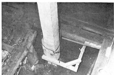
Fig. 16. Foot of standard column
