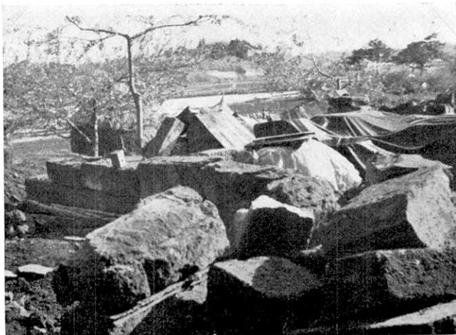
(c) Collapsed storehouse made of stone.
