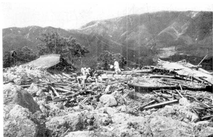
Fig. 10. The collapsed temple (wooden building).
