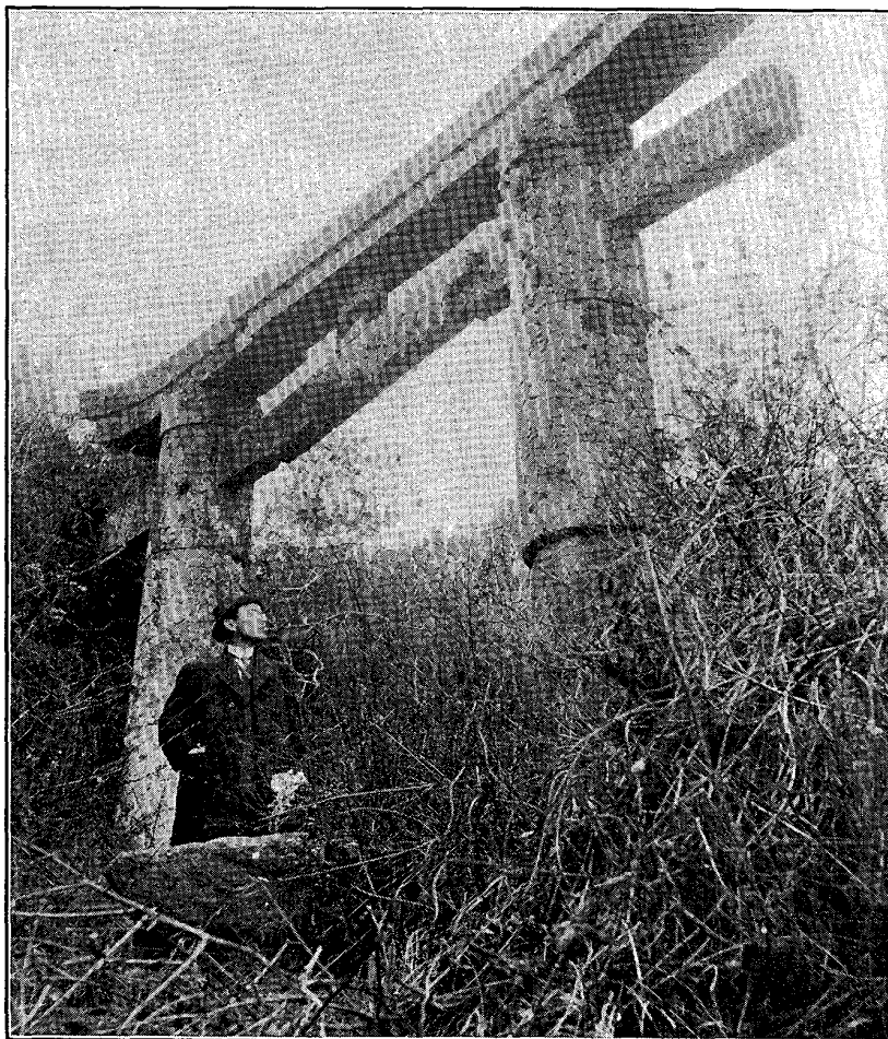
Fig. 2. The dislocated Torii near Asabataké.
