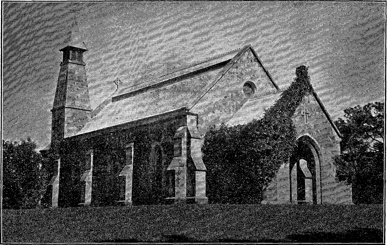
Fig. 24. A Church, Shillong. (Before the earthquake.)
