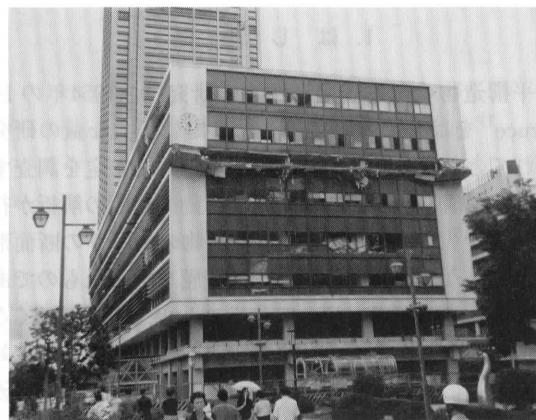
Photo 1 Local collapse at intermediate story of weak-column building
