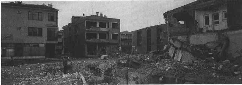
Destruction by Erzincan Earthquake, Turkey, 1992 (Photo by K. Meguro)
