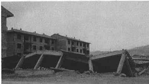
Photo 7 Totally collapsed apartment building [Yavuz Selim District]
