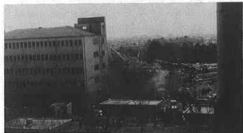
Photo 13 Collapsed Social Security Hospital [Inonu District]
