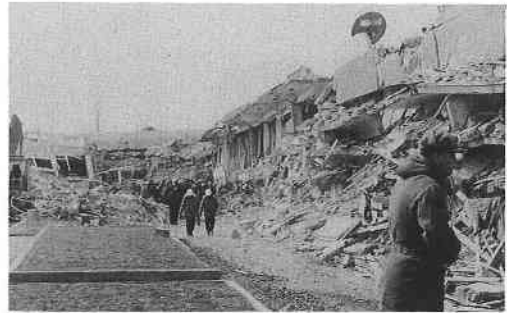
Photo 1 Totally collapsed Hotel Urartu (right) and Municipal Annex Building (left) [Kizilay District]
