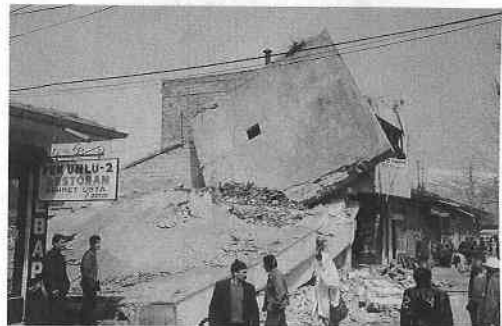
Photo 2 Totally collapsed residential building [Kizilay District]
