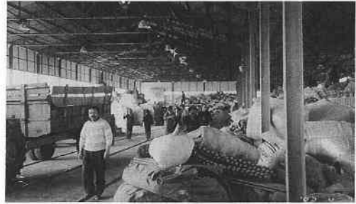
Photo 19 Interior of the warehouse
