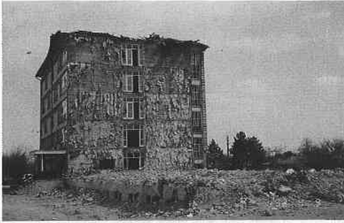
Photo 5 Collapsed State Hospital
