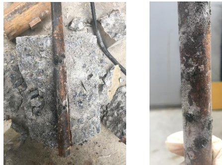
(a) Corroded bar removal
