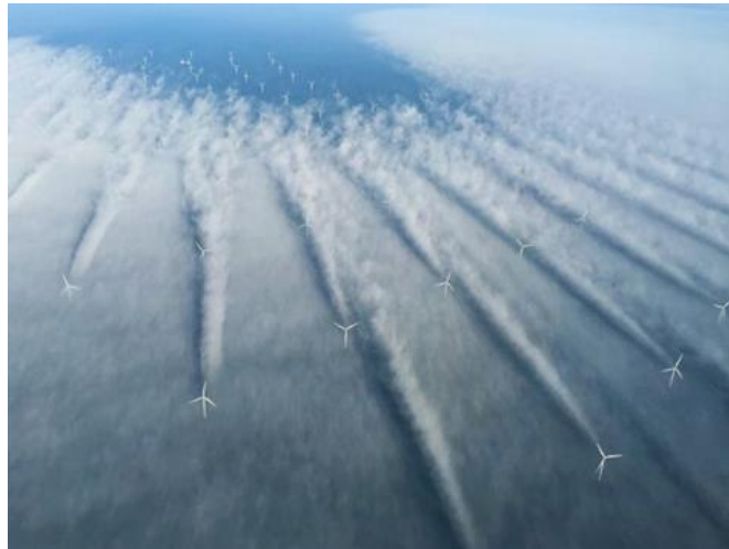
(a) Offshore wind farm, Horns Rev2, Denmark
