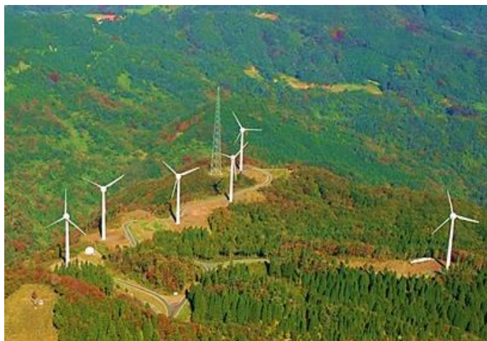
(c) Wind farm in mountainous areas, Taikoyama, Japan
