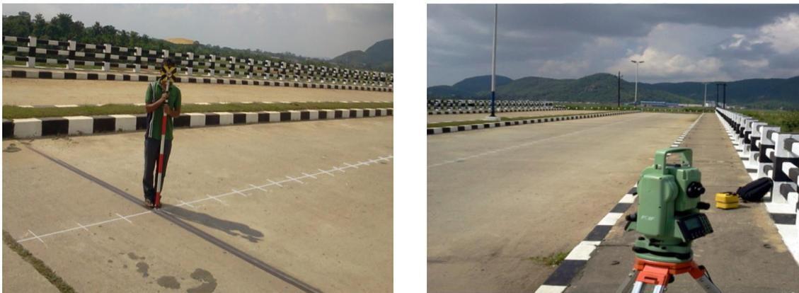
Fig. 1-3. Measurement using a total station (Lalthlamuana, 2015)
