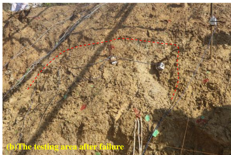
Fig. 5-49 Images of the testing area before and after the slope failure
