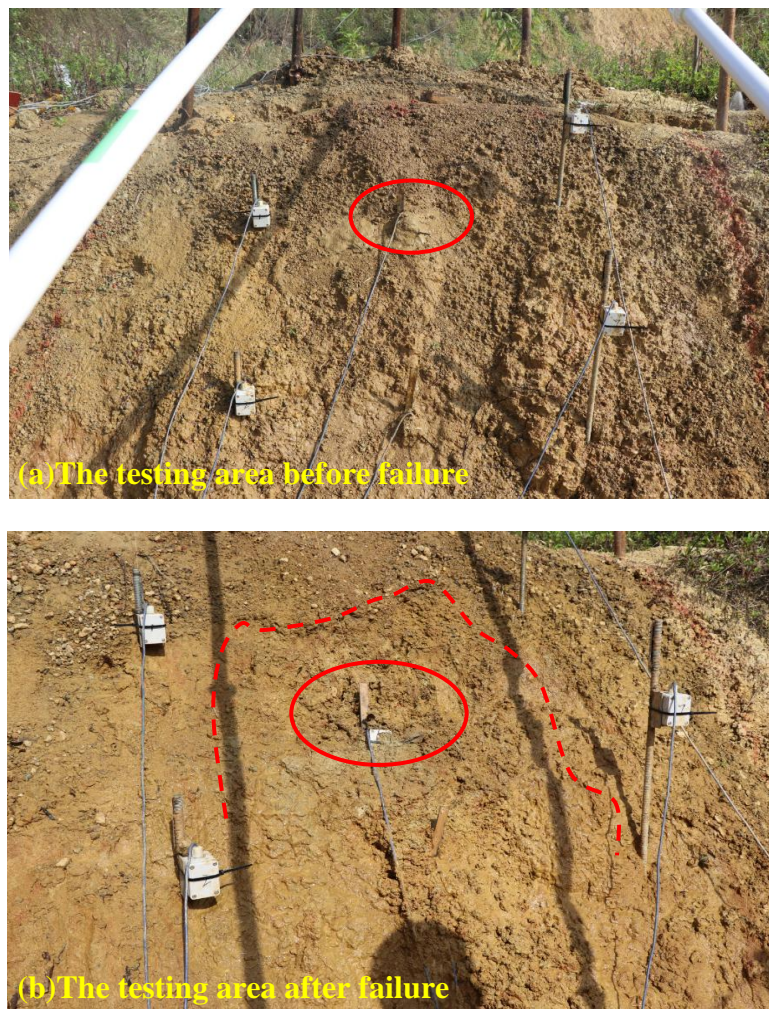
Fig. 6-92 Images of the testing area before and after the slope failure
