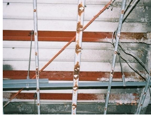
(b) Rust in ceiling frame
