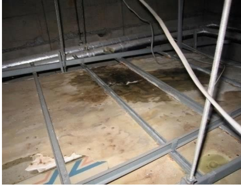
(a) Leaking of rain
