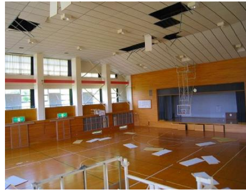
(d) Ceiling board fall by earthquake
