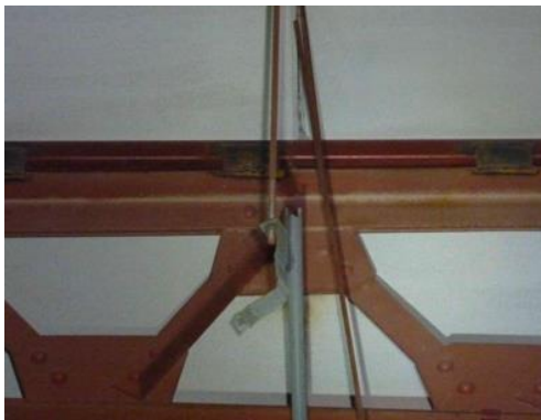
(c) Deformation of hangers
