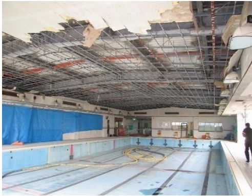
(c) Ceiling fall by dew condensation
