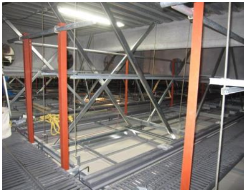
(c) Earthquake resistance enhancement
