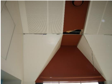
(b-2) Showcase 2: damaged ceilings from a nearer perspective, resolution: 2592×1944×3
