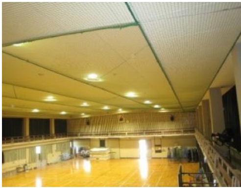
(a) Fall prevention net and wires
