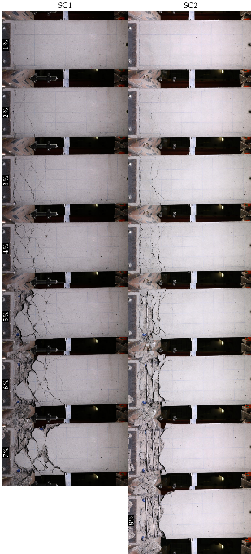
Figure D.25: Residual damage state at the end of cycle completion (SC1 and SC2)
