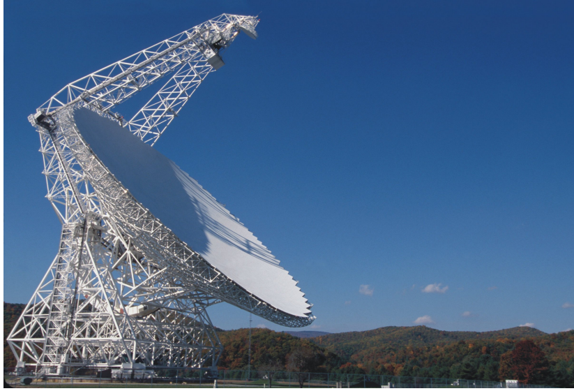
Figure 16. The 100 meter Green Bank Telescope.
