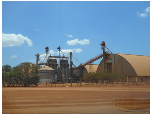
Figure 5-3: Large Scale Storage Facilities
