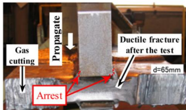
Fig. 9-18 Crack arrest in weld metal [29]
