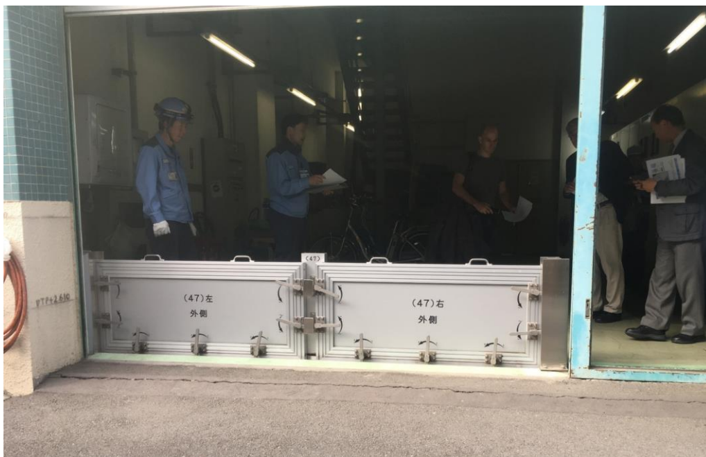
Figure 4.4. Countermeasures to prevent water intrusion into building, designed against the storm surge expected for an event similar to Typhoon Vera (T.P. +2.61 m) in Kiba Pumping Station
