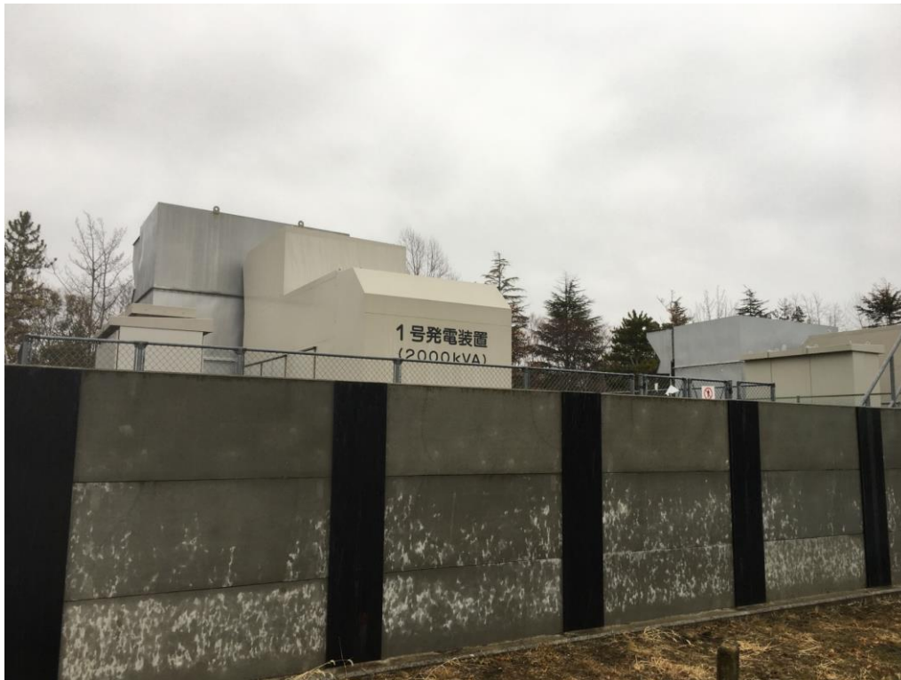
Figure 3.10. Electricity generation center of Sen-en WPC, showing flood prevention structures surrounding the facility
