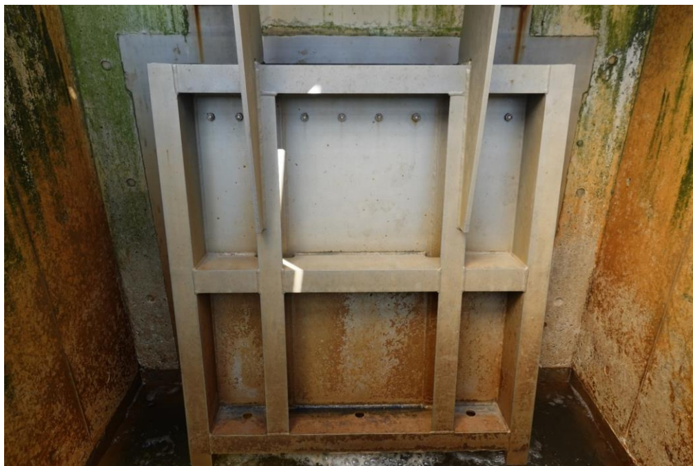
Figure 3.13. Discharge gate at Ishinomaki-Tobu WPC discharge channel. The gate can be closed to prevent seawater intrusion into the pipes.
