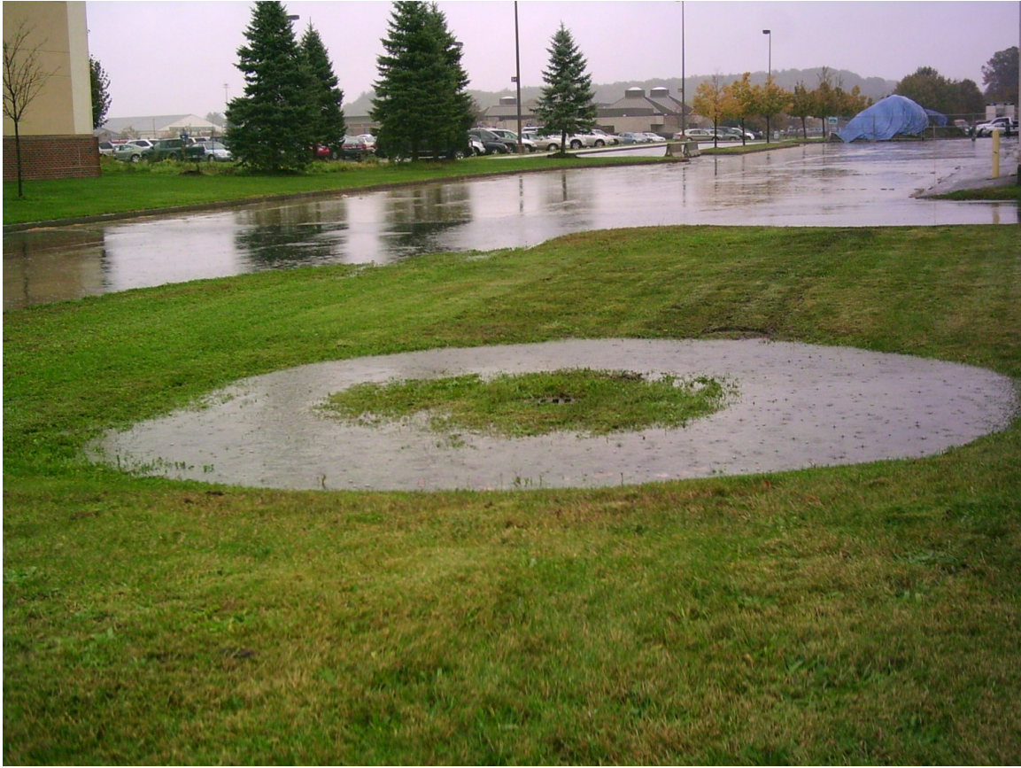
Figure 5-8. Bioretention BMP to capture and infiltration of runoff from parking lots (Pictures provided by Mr. Don Morris, USAF)
