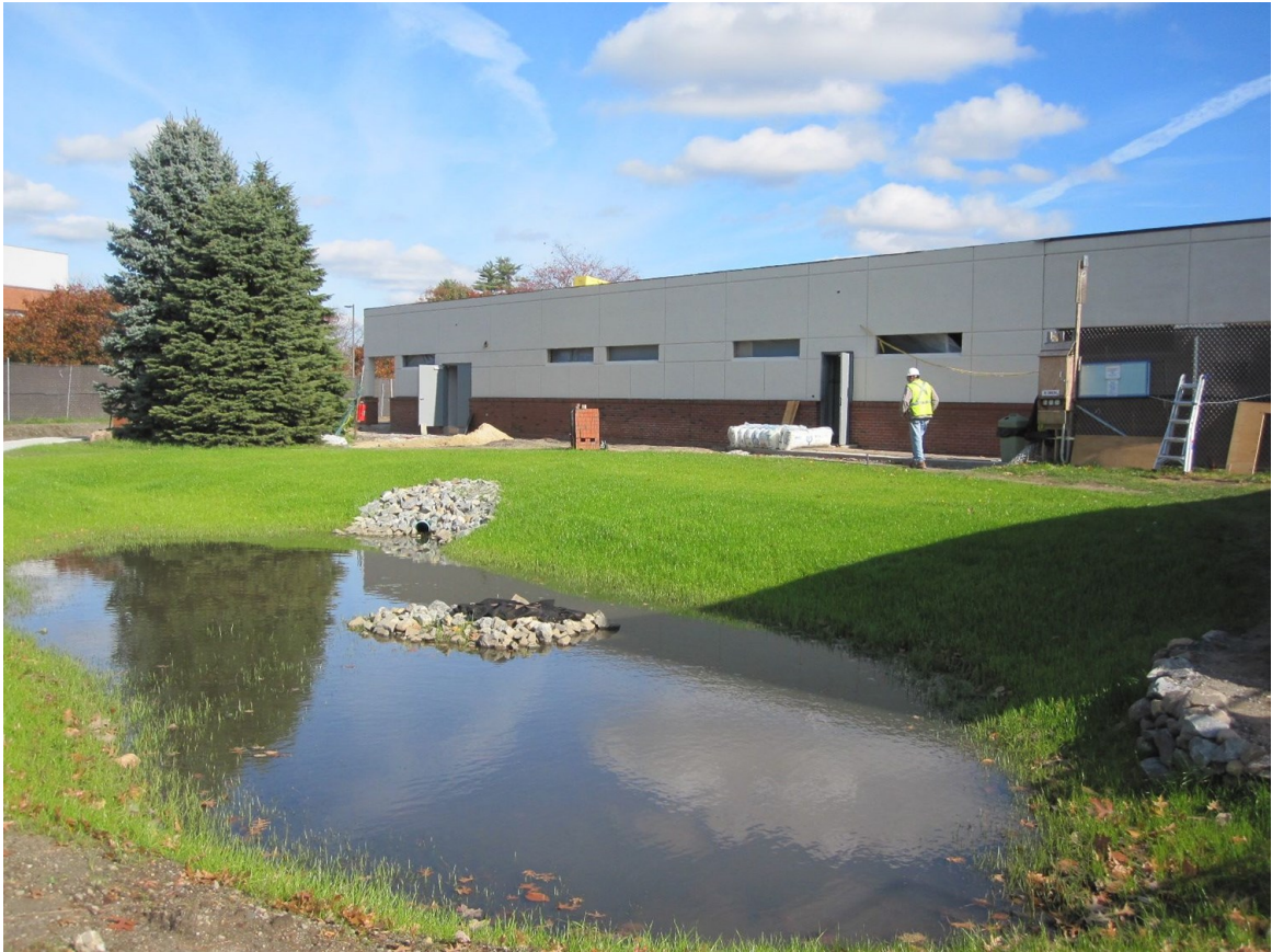
Figure 5-9. Extended Detention BMP to capture and detain for evaporation of runoff from parking lots (Pictures provided by Mr. Don Morris, USAF)
