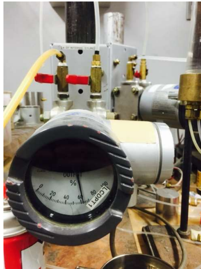
Figure 2.11: Low Capacity Differential Pressure Transducer (LCDPT)
