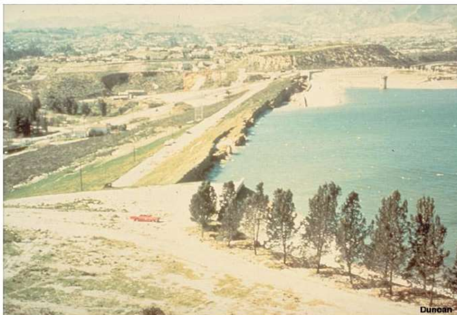
Figure 1.3: Slide head scarp general view (Photo courtesy Duncan)
