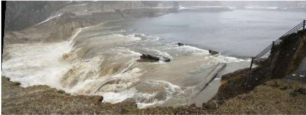
Figure 7. 2: Breaching and flooding of water after Tohoku earthquake (after Tanaka et al. 2012)
