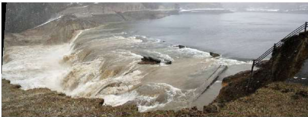
Figure 1.6: Breaching of Main Fujinuma Dam (Courtesy of Fukushima Pref.)
