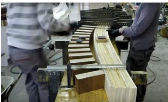
Figure 1-6. Steam bending wood with jigs and manpower (Making curved beams, 2017)
