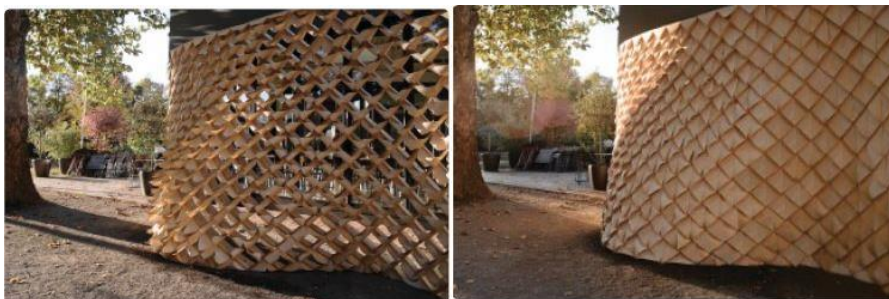
Figure 5-6. FAZ summer pavilion, openings responded to the weather changes. (Menges & Reichert, 2012)
