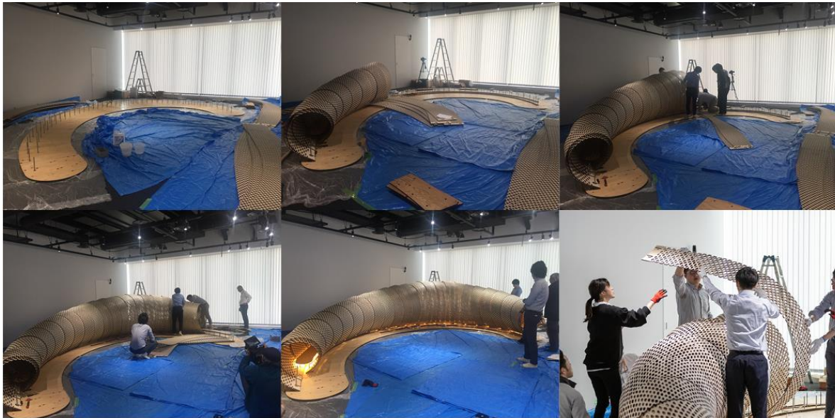
Figure 4-21. It took only one day to roll up all the spiral pieces.
