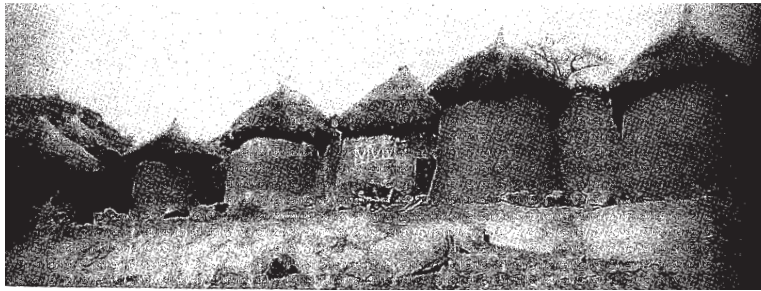
Figure 2.2. Mesakin, Nuba Mountain, Southern Sudan, 1955, mud houses on a mud platform (Denyer, 1982, p. 12)
