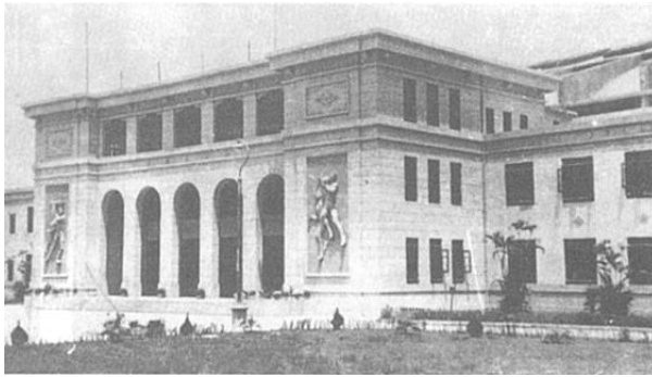
Fig. 2-8. Guangzhou Gymnasium by Lin Keming, 1955—57 (Zhou, 197)
