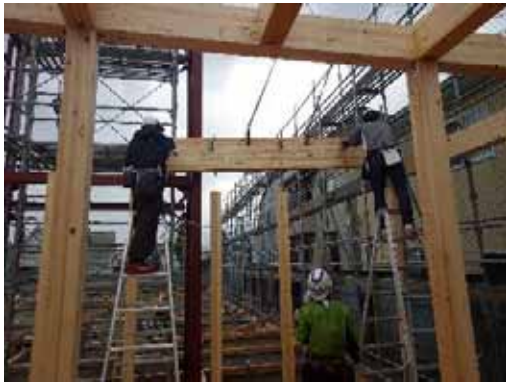
2F 床梁_揚重取付
