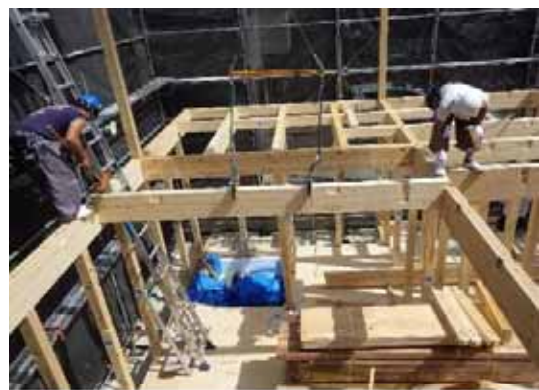
2F 床梁_揚重取付
