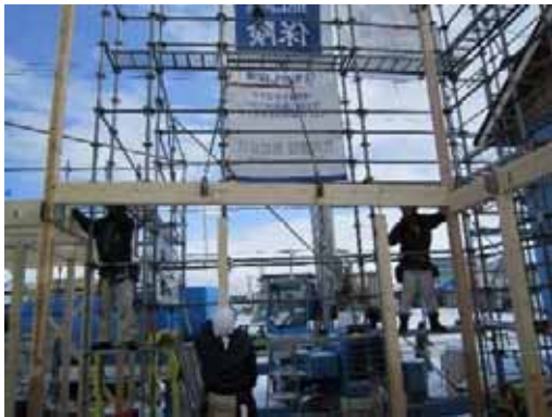
2F 床梁_揚重取付
