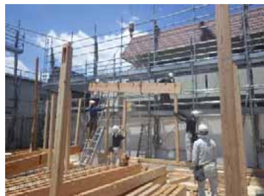
2F 床梁_揚重取付
