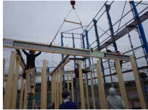
2F 床梁_揚重取付
