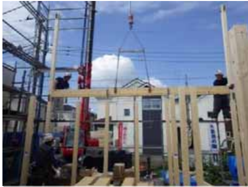
2F 床梁_揚重取付
