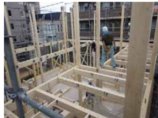
2F 床梁_揚重取付
