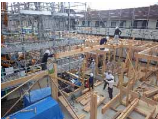
2F 床梁_揚重取付 (2)
