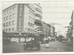
Photo 2. Outer Appearance of the Favoriten Bank.
