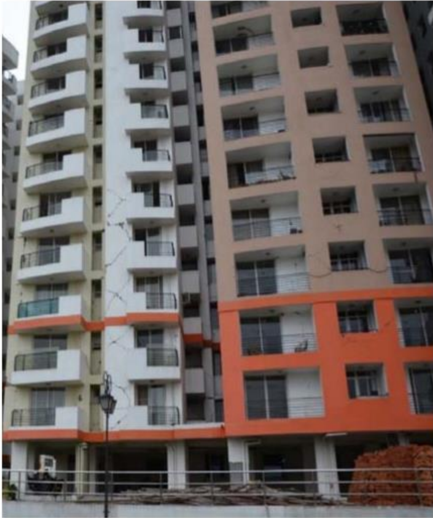
Damage and cracks in the high-rise buildings
