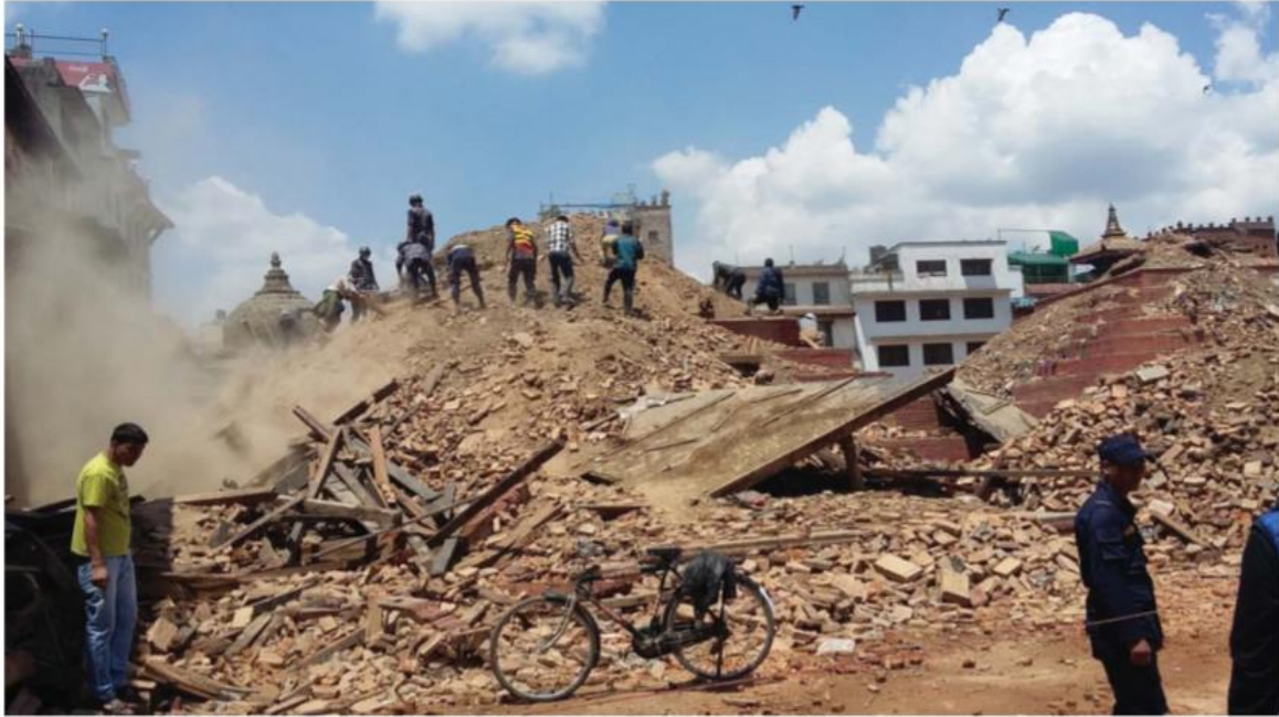
Damage observed in the historical mounements at Kathmandu durbar square
