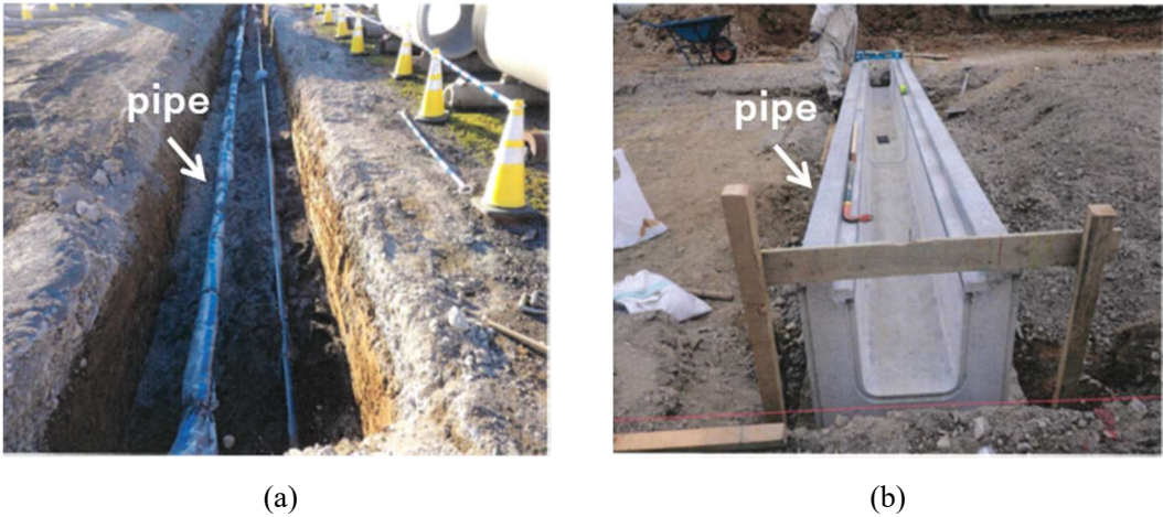
Fig. 2.12 Construction of pipe site (a) metal pipe (b) concrete pipe
