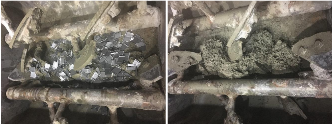
Fig. 4.3 Addition of steel fibers during the concrete mixing process.
