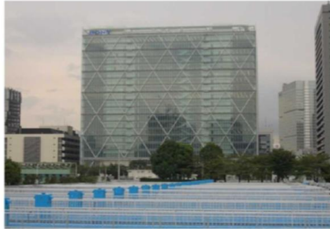
Figure 1- 8 Sony city building [25]
