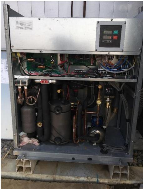
Figure 3. 19 Heat pump unit imported into the circulating water temperature control system
