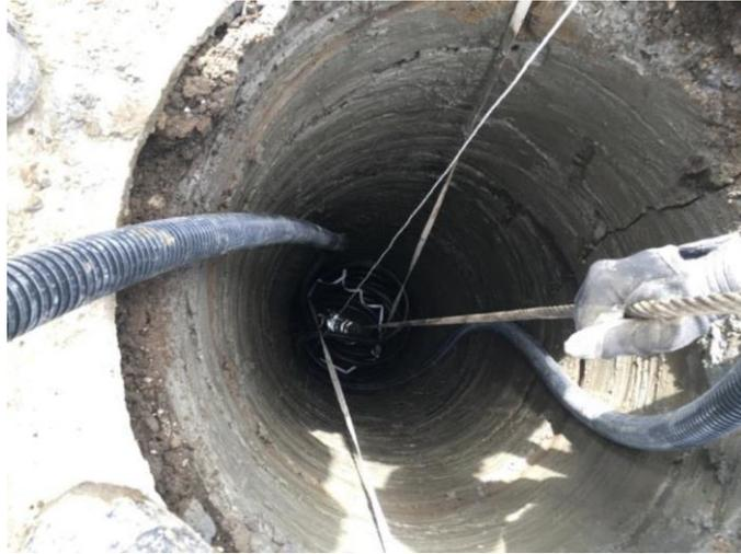
Figure 3. 26 Inlet/outlet connection piping with GHX coil
