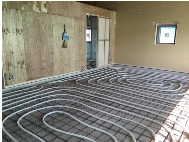
Figure 3. 31 RE house floor heating pipe system. (floor mortar & before floor tile finishing)
