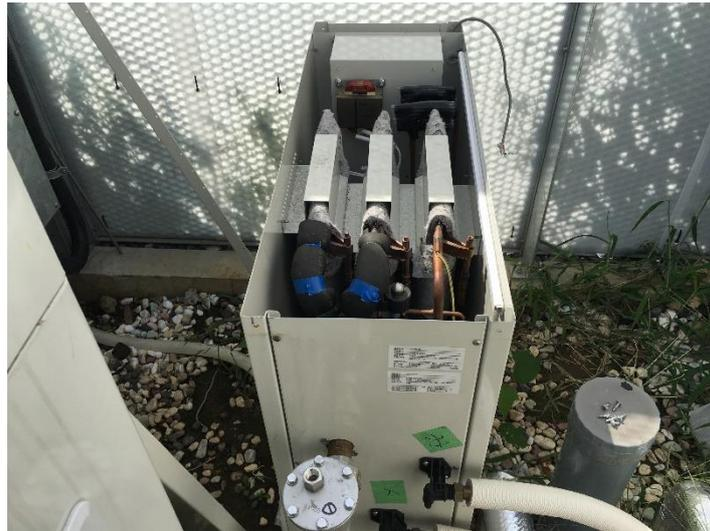
Figure 3. 42 Top view of water source heat pump for domestic hot water supply.
