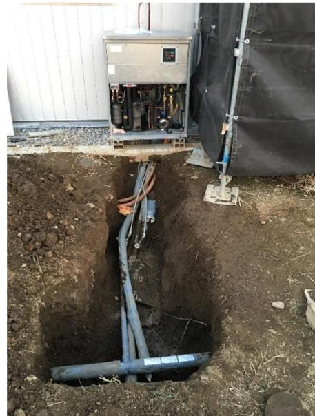
Figure 3. 20 Pipe connection with the water loop and sky source heat pump
