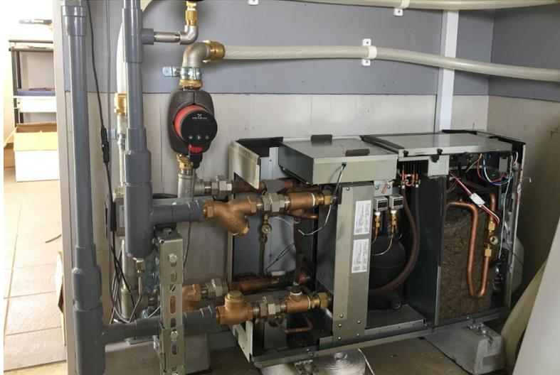
Figure 3. 3 Circulating pump set with heat pump together
