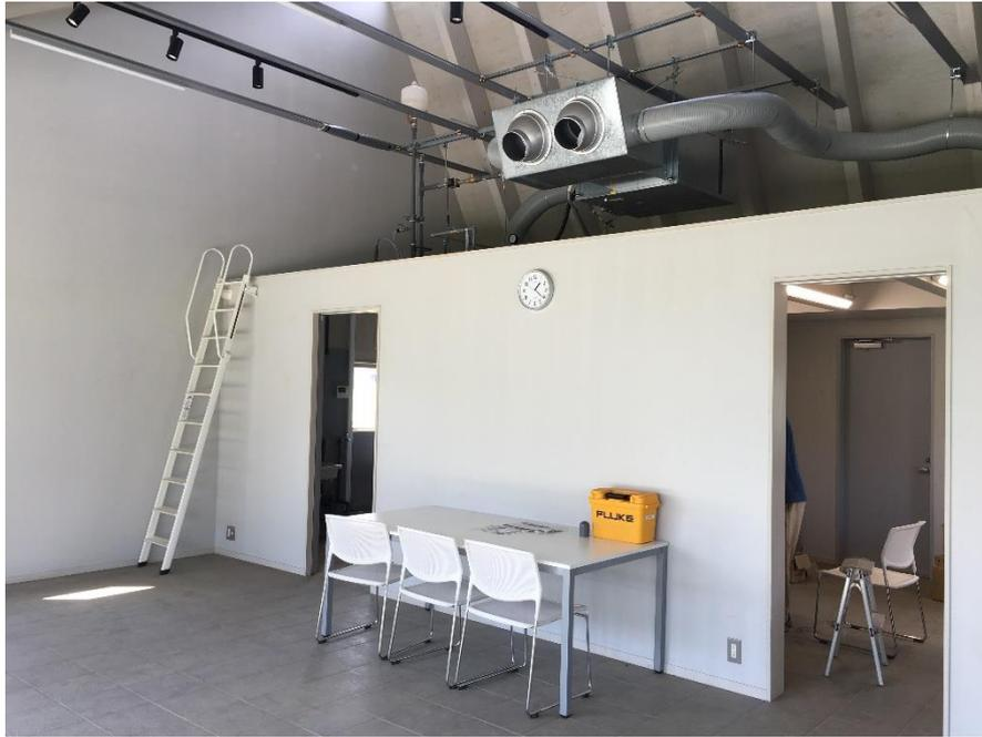
Figure 3. 37 Installation in the loft of the RE house and connected the duct and blowout nozzle.
