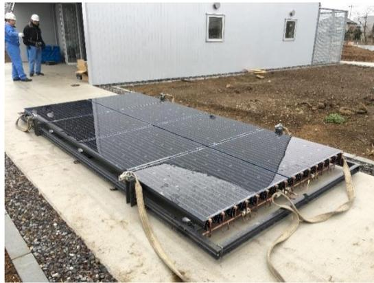
Figure 3. 10 The outdoor panel of sky source heat pump.
