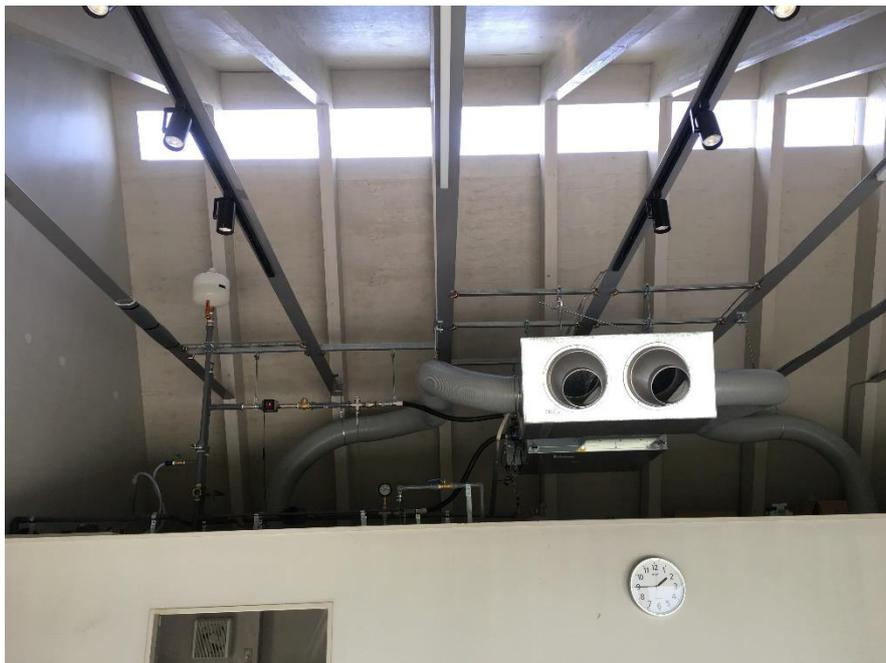
Figure 3. 38 The heat pump for air conditioning set on the loft and duct
