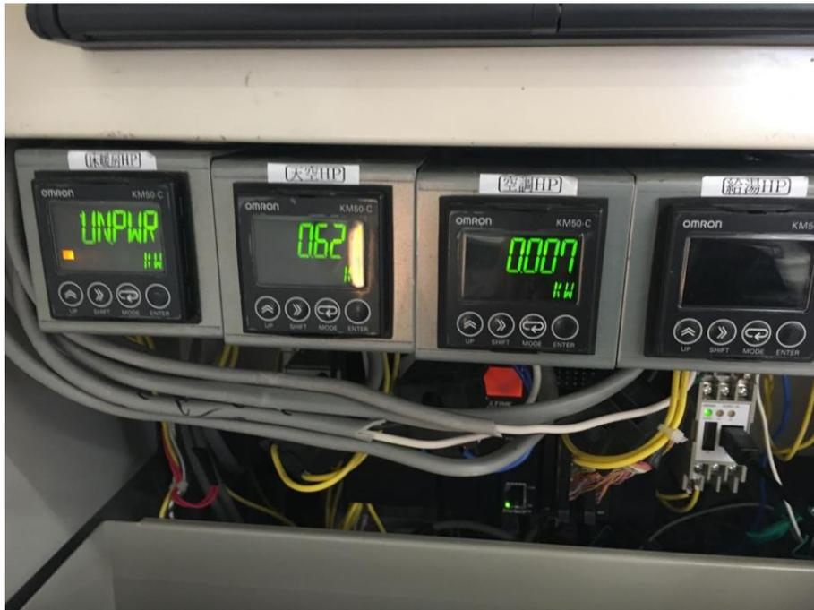
Figure 4. 11 Measurements of the energy consumption of each heat pump unit.
