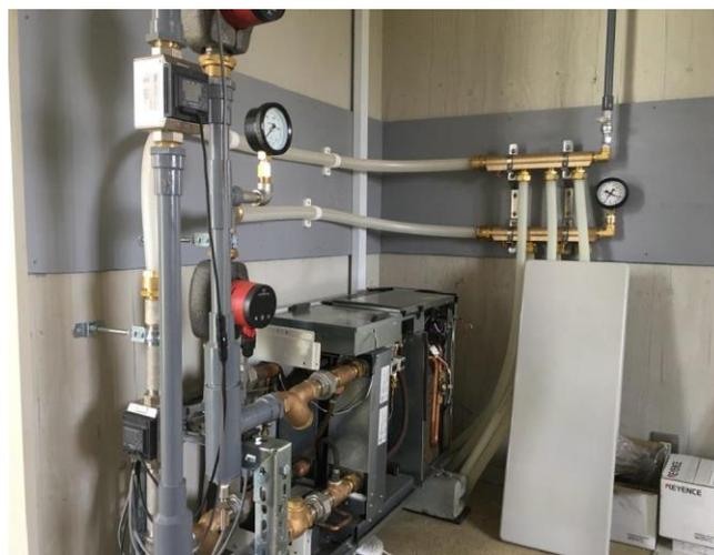
Figure 3. 32 Water source heat pump for floor heating installed in RE house.
