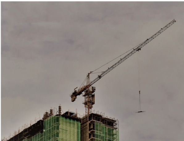
(c) Tower crane [60]
