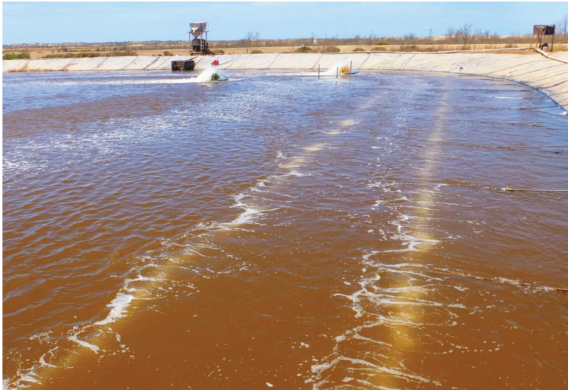
Figure 2.1 Diffused air aeration system [19].
