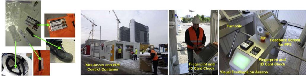
**Figure 1.3: A passive RFID portal for on-site PPE management proposed by Kelm et al.**
