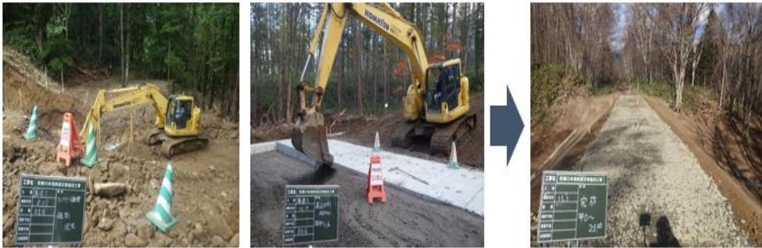
Figure 7. Excavation and embankment operation process
