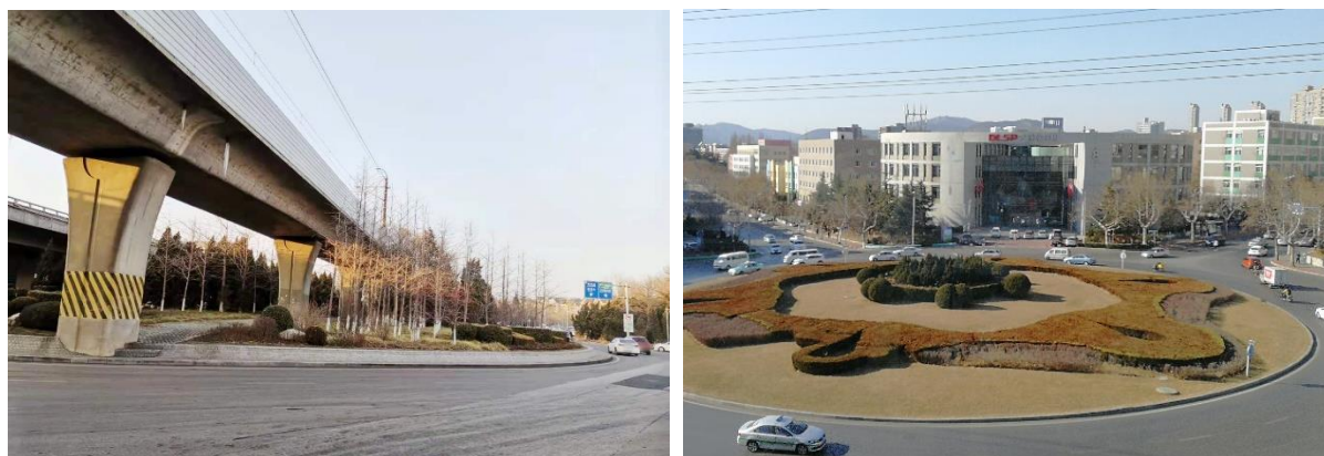
Fig. 6-10 RS&Rs constructed in 1980s (left, Haida Square) and 2000s (right, Shuma Square) in Dalian (Photos by author)
