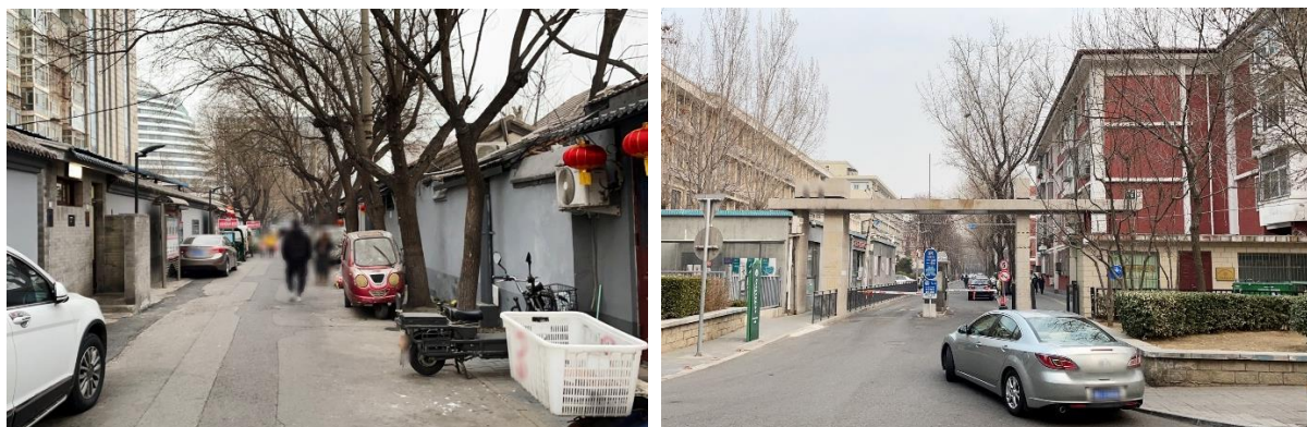
Fig. 4-13 Branch road in city plan but with width resemble Hutong (left, Dafangjia Hutong) Branch road in residential community (right, Hepingjiayuan Community) (Photos by author)
