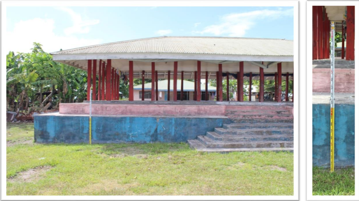
Figure 6.3 Modern traditional structure with an elevated cement foundation of about 165 cm
