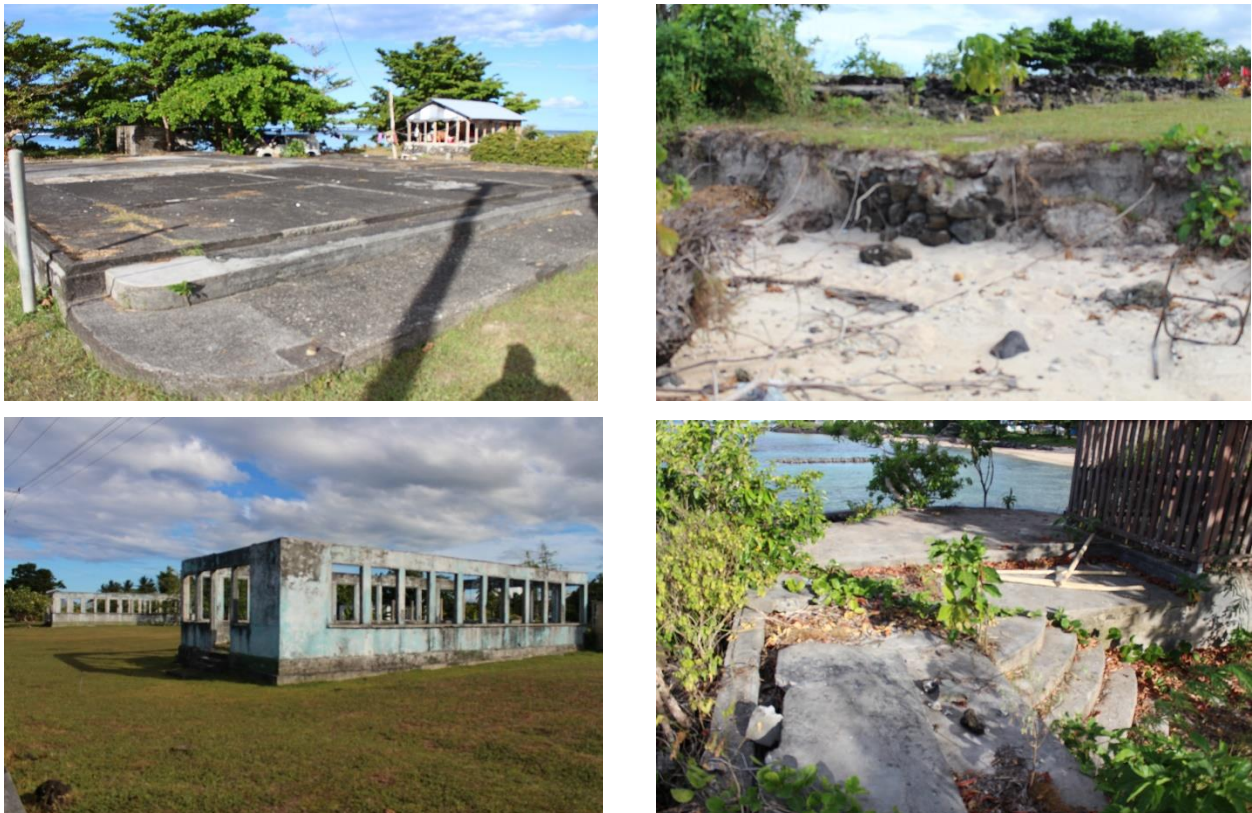
Figure 3.9 More images of abandoned areas in Fagamalo village. Former National district hospital (top right), Eveni, a private retailing company (bottom right), Foundation unearthed with beach erosion (top left) and entrance to was formerly a school (bottom right)
