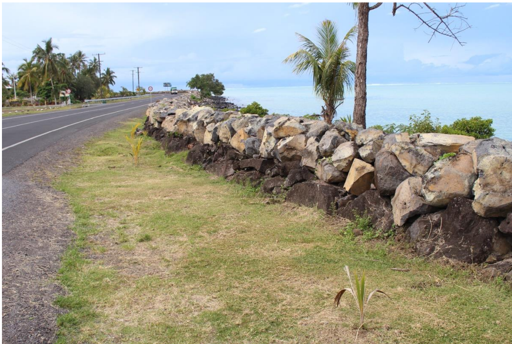
Figure 6.1 Newly elevated national road along the coastline of Upolu Island, and elevated coastal rock revetment.
