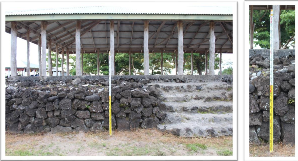
Figure 6.4 Modern traditional structure with a stone foundation elevation of about 150cm
