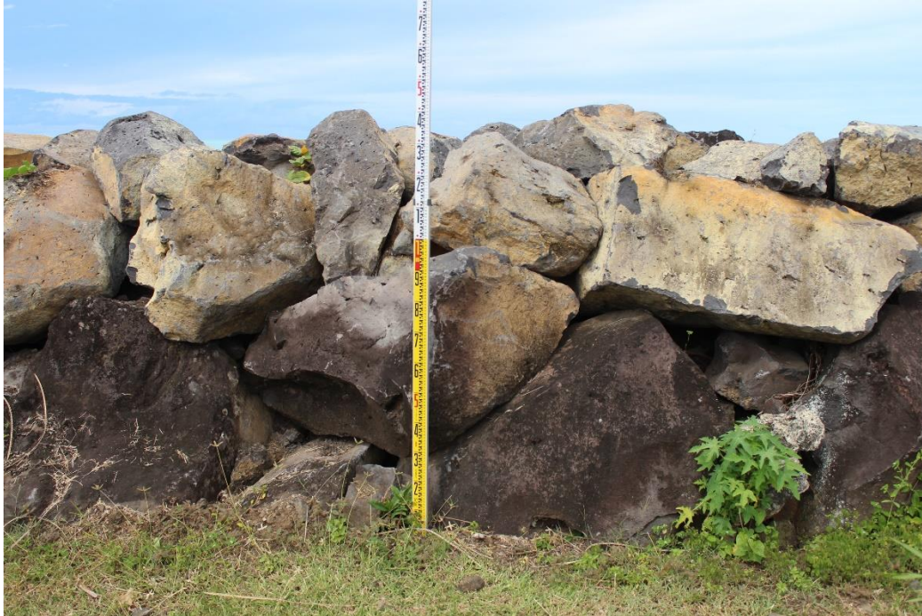
Figure 6.2 Height of the revetment crown.
