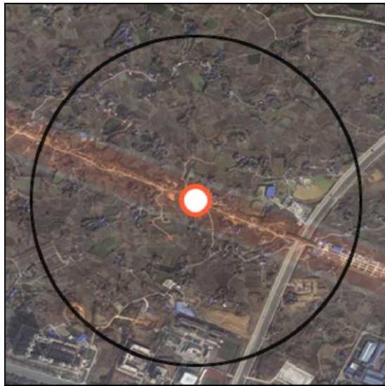
Figure4- 5 Line 2 Lianshanpo Station Construction Permission in 2012
